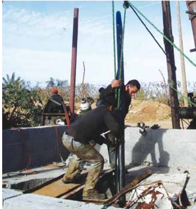
In the process of rehabilitating one of the wells.
