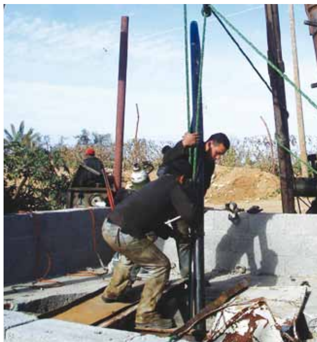
In the process of rehabilitating one of the wells.
